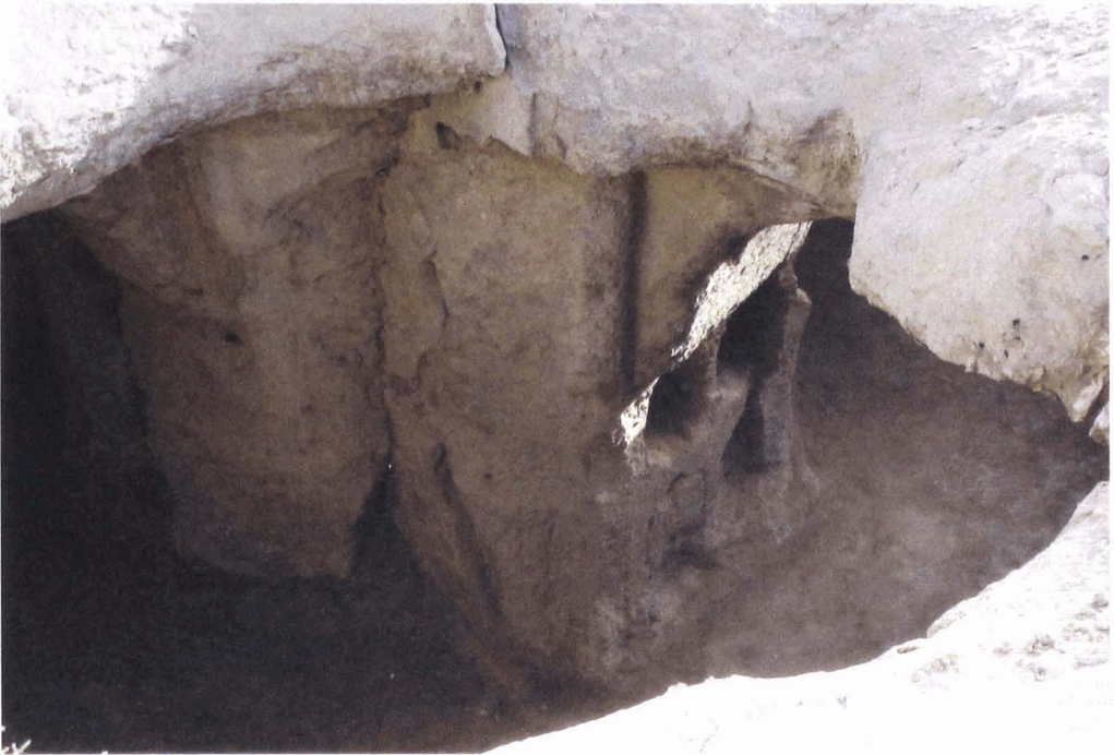
10.5 Mihrī Temple/Imānzāda Ma‘šūm: pillar of chamber no. 3 seen through one of its four collapsed domes. Photo: A. Azad.
