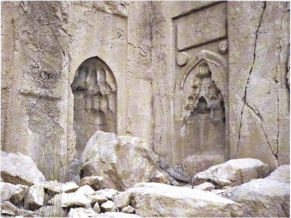
10.10 Dāsh Kasan (Qonqor Olong): set of adjacent mihrābs in the south-western corner of the façade. Photo: A. Azad.
